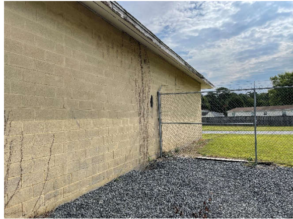
8. South Side – Fence encloser and hole in CMU
