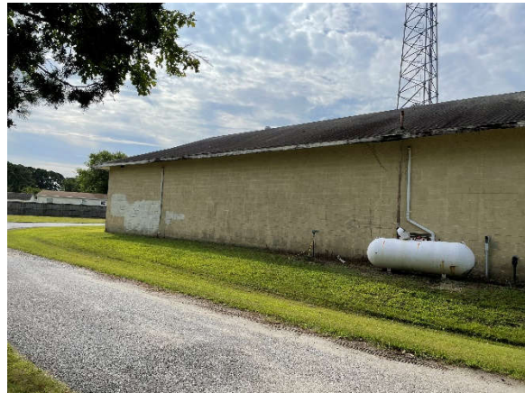
4. North Side – Deteriorated Fascis, missing gutter and grading
