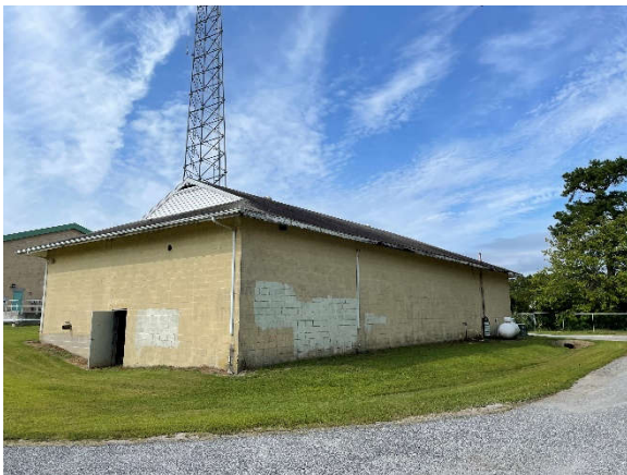
5. East/North Side – Deteriorated Fascia and grading.
