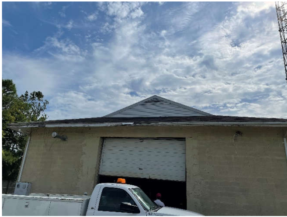
1. West Side – Missing gutter and deteriorated fascia.
