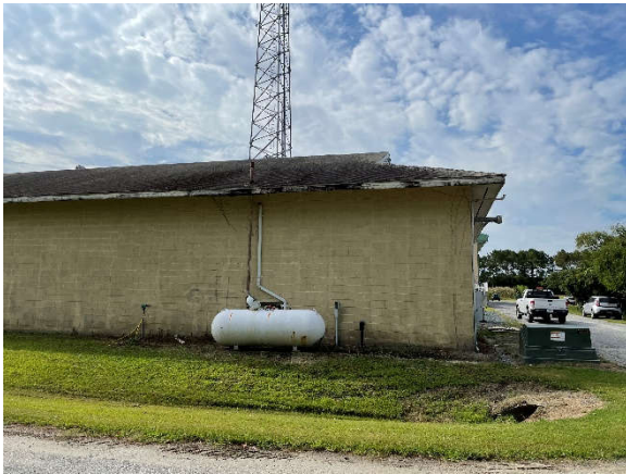
3. North Side – Existing propane tank, deteriorated fascia, missing gutter and grading.
